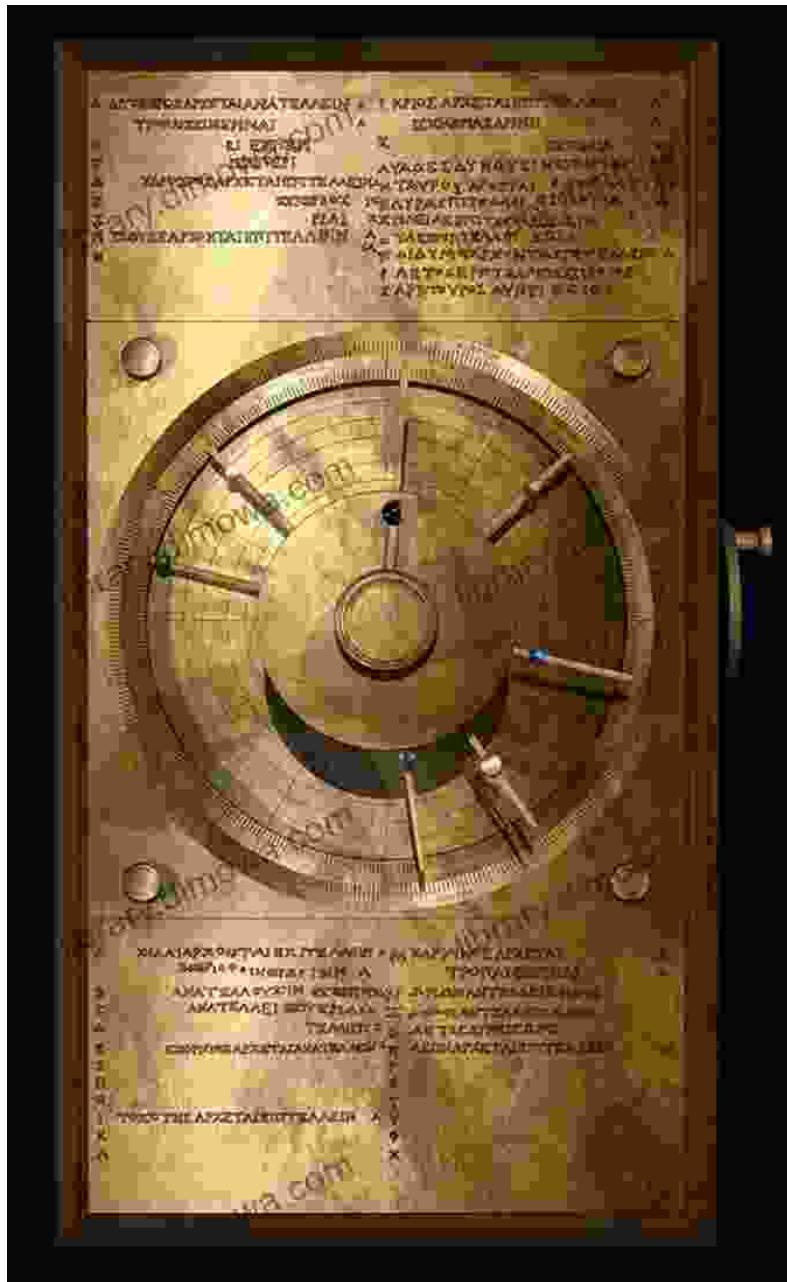
The Antikythera Mechanism, discovered in a shipwreck in 1901, stands as a testament to the advanced engineering skills of the ancient Greeks. This remarkable device, dating back to around 100 BC, was capable of accurately predicting astronomical events, performing complex calculations, and even displaying the positions of the sun and moon. Its
